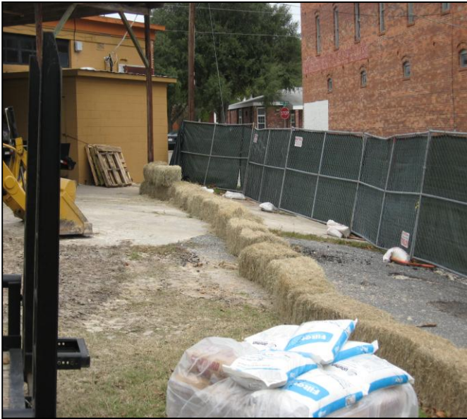
Photograph 7: Silt fence and hay bales are used for stormwater control.
