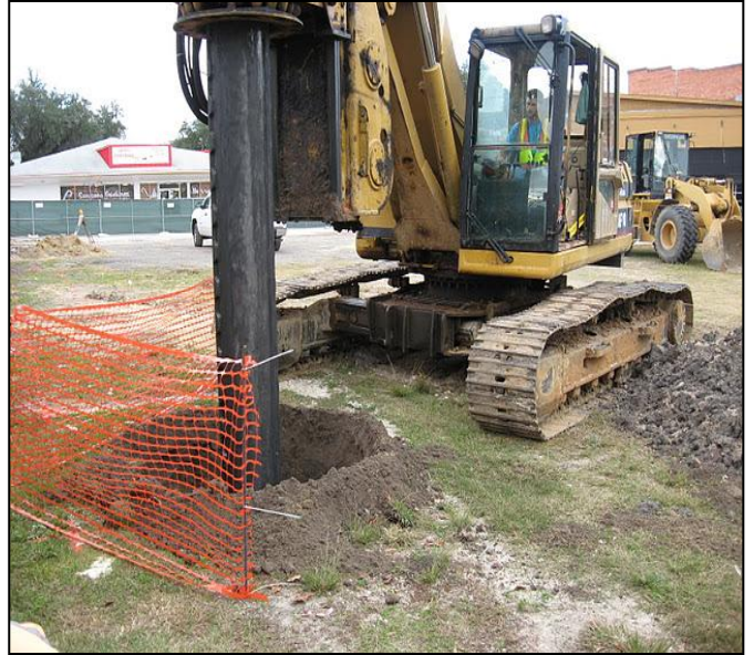
Photograph 2: Each boring was drilled to 20 feet with a traditional LDA rig with 5-foot dia auger.
