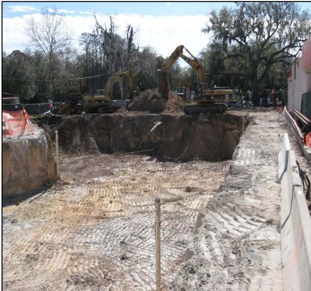
Photograph 3: five inch diameter dewatering wells are seen close and far.
