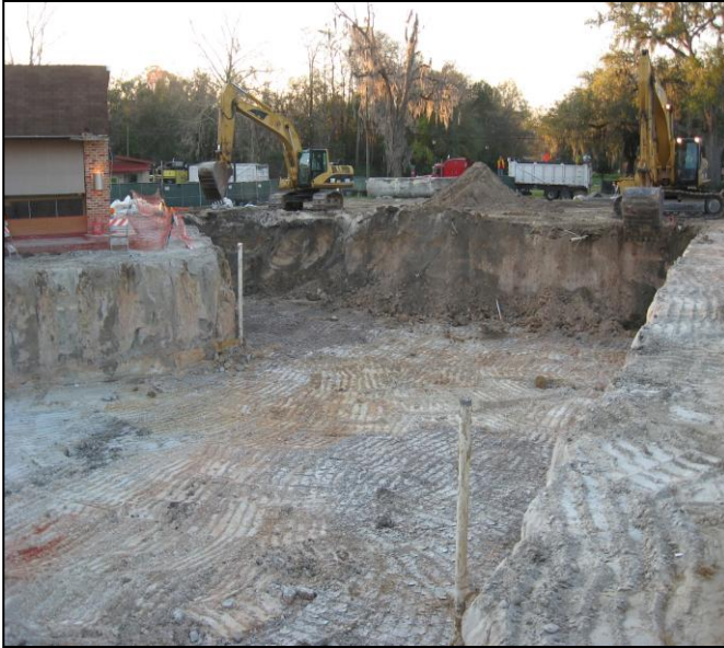
Photograph 5: Shadd excavation approximately 2/3 of the way back to 10 feet bls.
