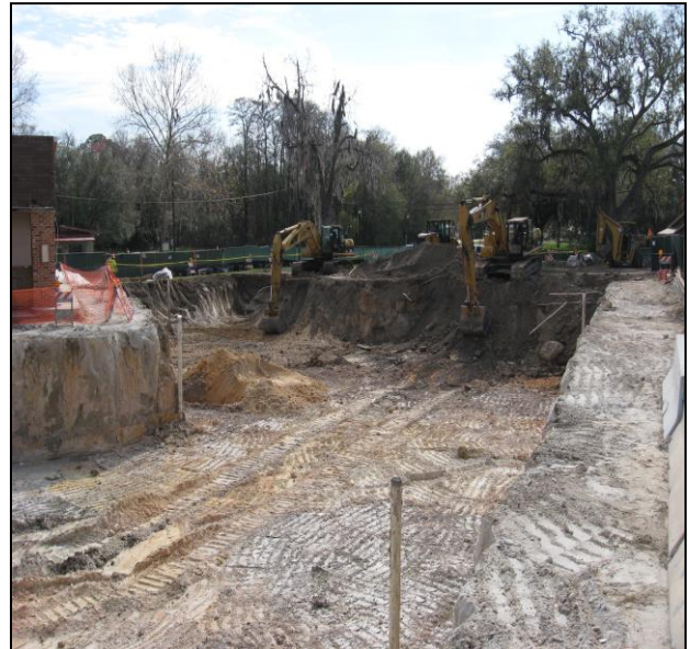
Photograph 2: Dewatering manifold is shown to right along jersey barriers.
