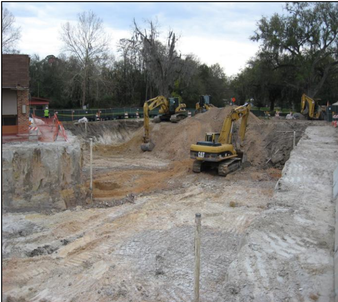
Photograph 7: Shadd excavation, showing sloping in southeast side of excavation.
