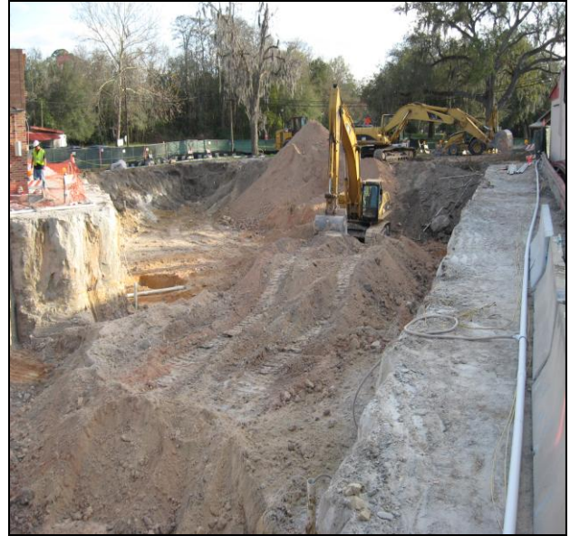
Photograph 2: Dewatering manifold is shown to right along jersey barriers.
