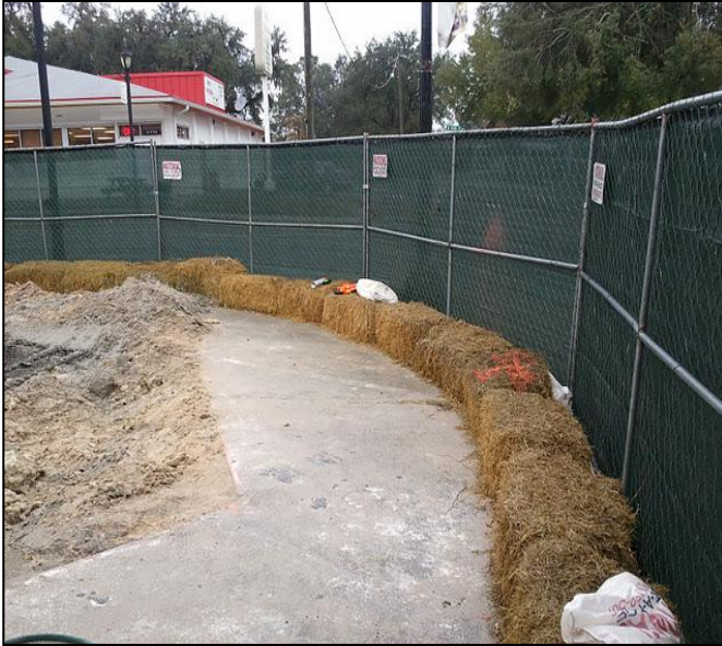
Photograph 5: Stormwater controls at the corner of Main Street and 2 nd Avenue. .
