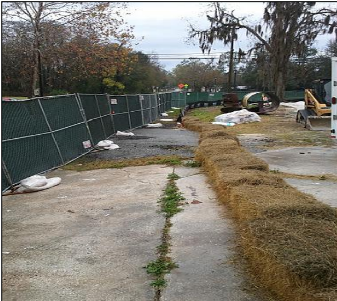
Photograph 7: Stormwater controls on 2 nd Avenue.
