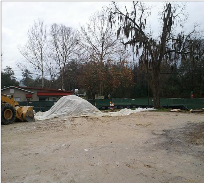
Photograph 3: Contaminated soils not directly loaded and removed were covered with plastic.
